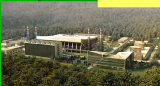
Base stations for heat supply – gas powered boilers
