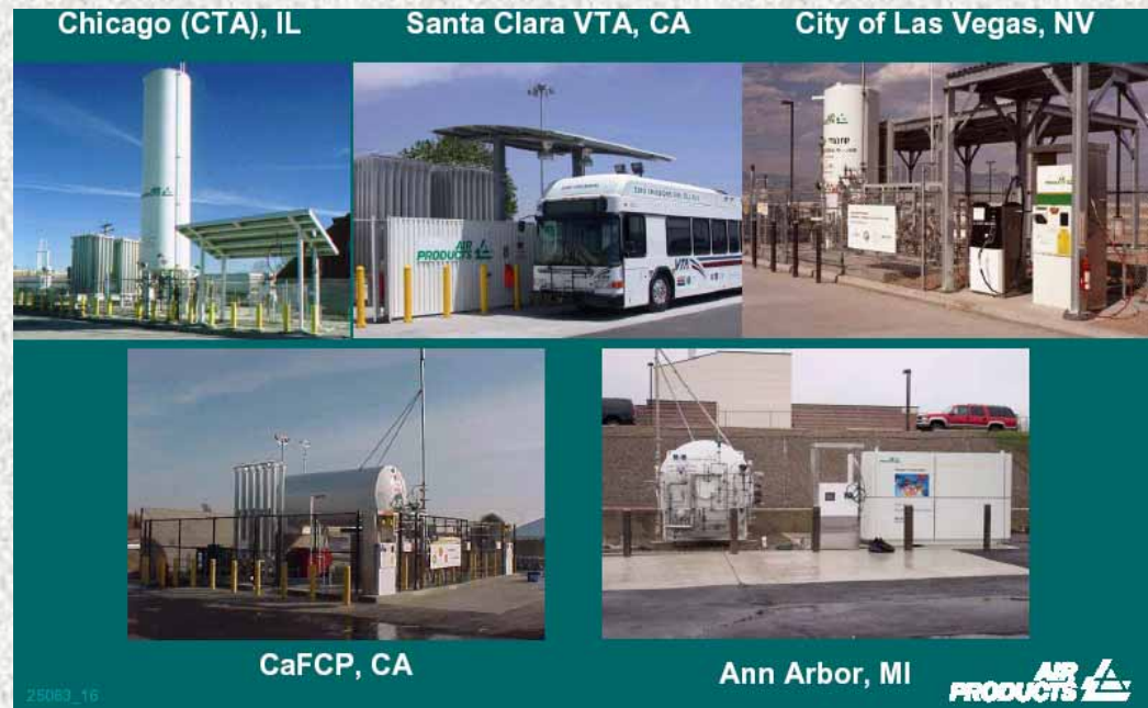
Liquid hydrogen fueling stations
