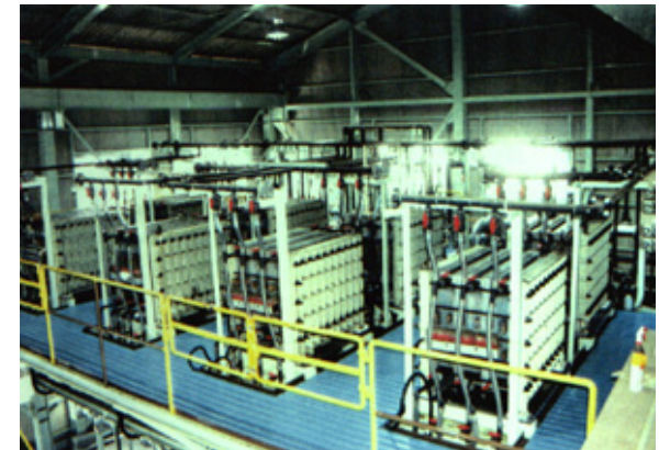
Kashima-Kita power plant (Japan)
